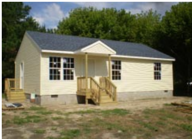
IPR Replacement House
