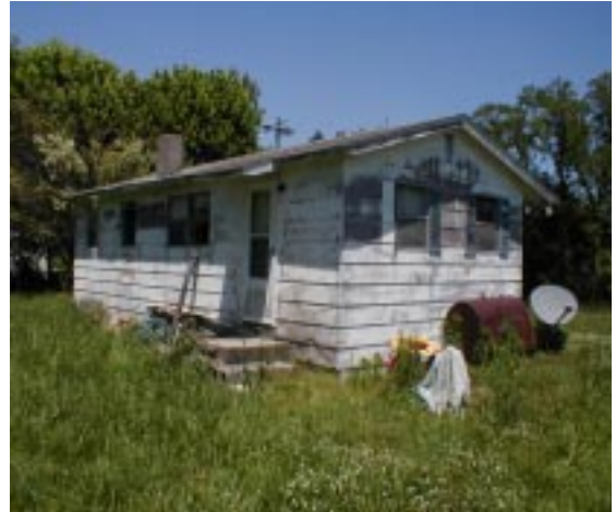
House lacking indoor plumbing
