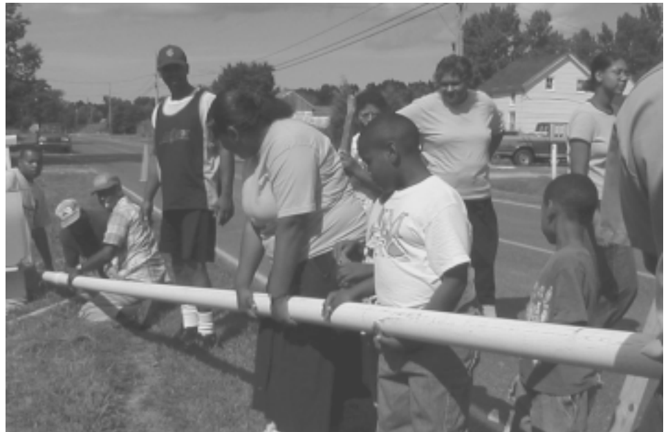
Community residents install wastewater pipelines in Makemie Park
