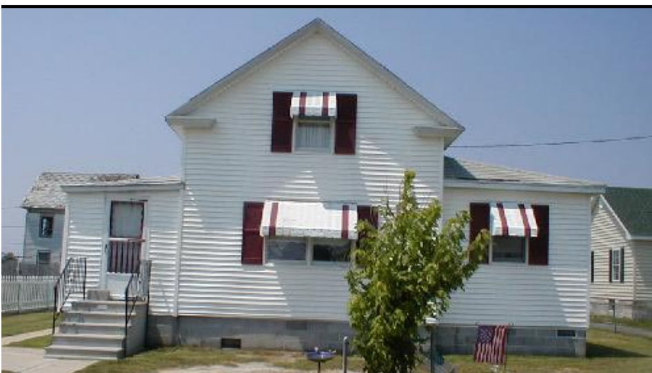
Home Elevated Above the Hundred Year Floodplain on Tangier Island by a FEMA Mitigation Grant
